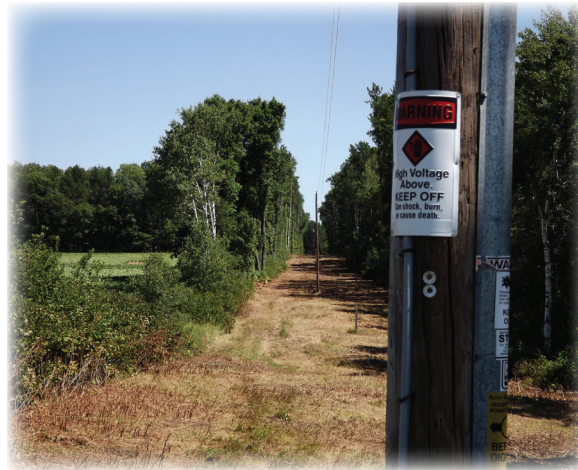
A clear right-of-way improves power quality, reliability and safety.
